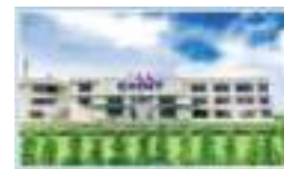
Thailand Solar Power Production Base
